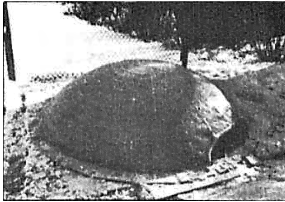
Figure 12: Dome made of ice reinforced with fibreglass [3].
