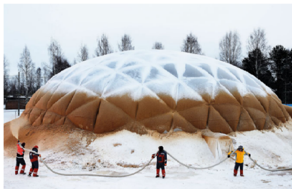
Figure 14: Making of a pykrete dome [9].
