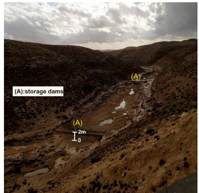
Fig. 11. . Location of sediment storage dams.
