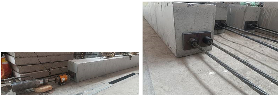
Fig. 6. Prestressing tendon tensioning: a) Holding a load, b) After tensioning
