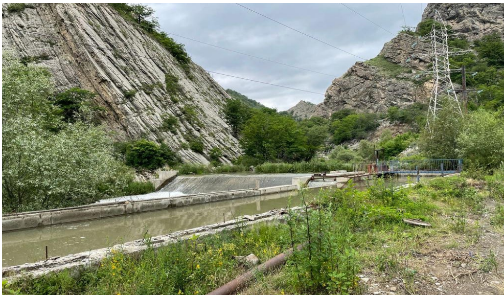
Fig. 4. Water intake structure for small hydroelectric power plants Source: developed by the author
