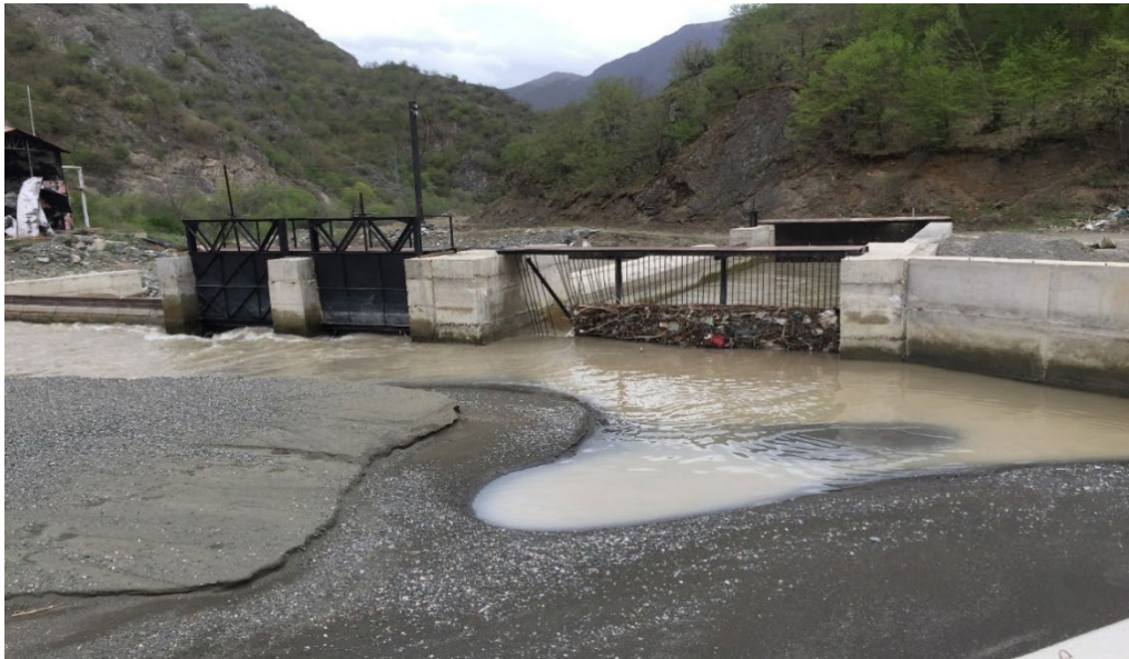
Fig. 1. Water intake structure for small hydroelectric power plants of the Kalbajar district Source: developed by the author
