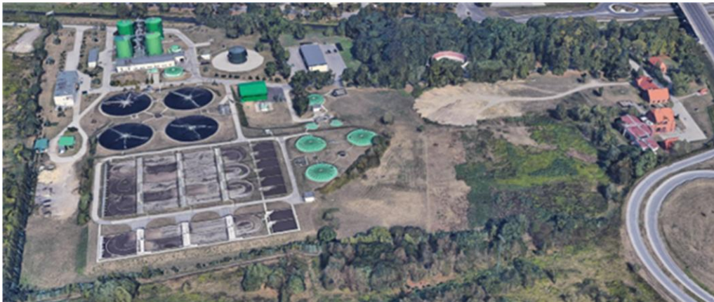
Fig. 4. Central Sewage Treatment Plant of Gliwice (source: Google Earth).
