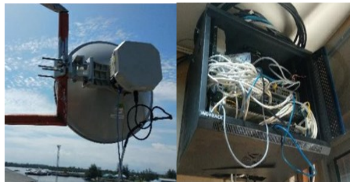
Fig. 2. Radiolink (a) ODU (b) IDU
