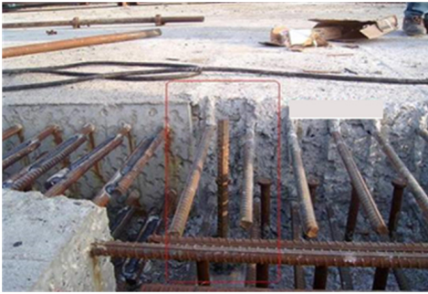
Fig. 17. Positioning points for main girder elevation measurement
