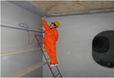
Fig. 14. Strain sensor installation diagram
