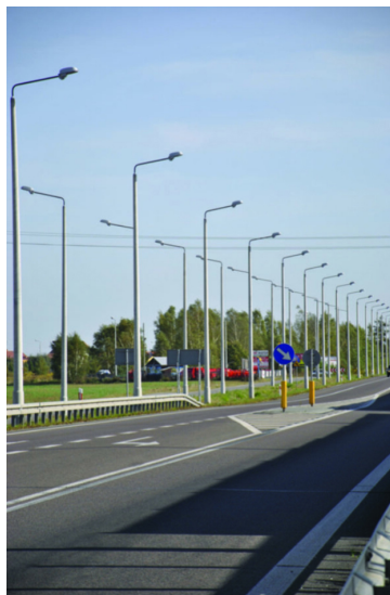
Fig. 1. Composite circular GFRP lighting poles [2]
