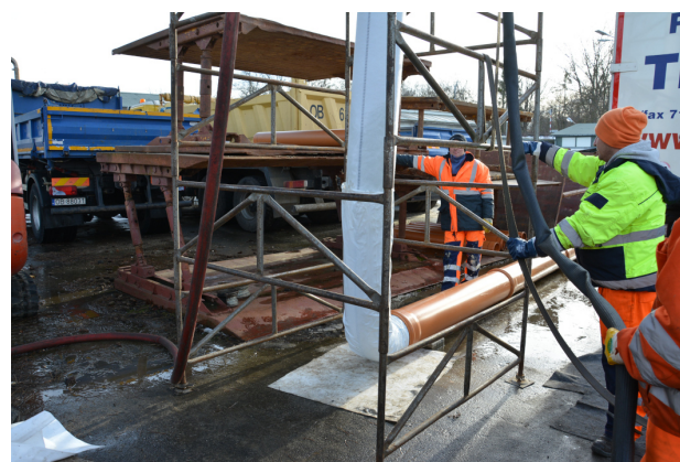
Fig. 5. Inversion tower and the insertion of the CIPP lining into the PVC pipe
