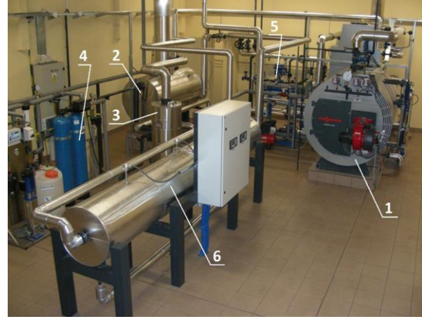
Fig. 5. General view of the laboratory station: 1 - steam boiler, 2 - deaerator, 3 - sludge expander, 4 - water treatment station, 5 - reduction station, 6 - steam header.
