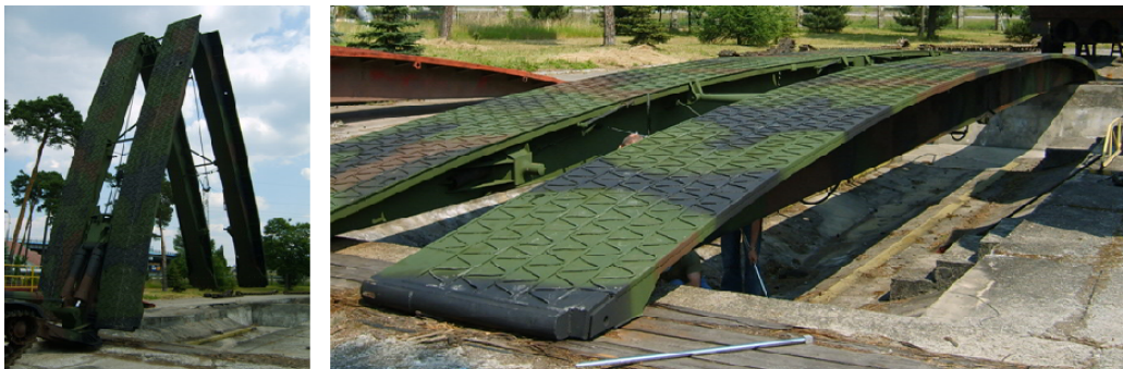
Fig. 1. A view of the tested BLG bridge during the deployment process, the stand intended for tests and examinations of BLG bridge that is deployed to a crossing position
