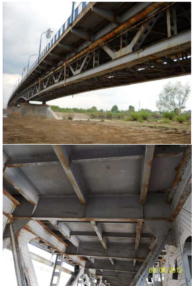
Fig. 1. The existing riveted truss bridge and its deck system
