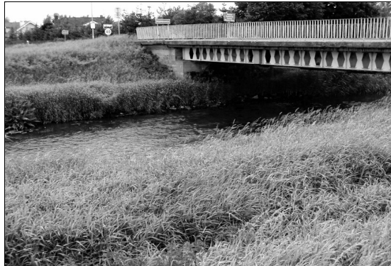
Fig. 3. The River Widawa, Krzyzanowice station, Spring 2012 [Photo R. Kasperek]
