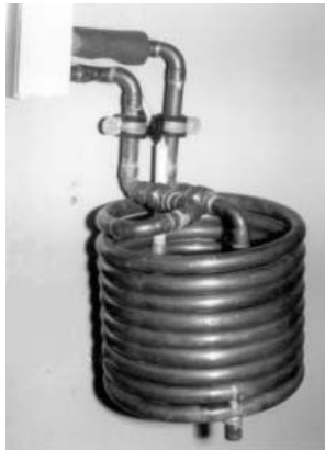
Figure 10. Cooler – heat exchanger; takes heat from the heat-carrier (without a tank-container).
